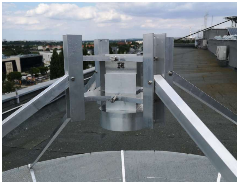
Fig. 1.3 Feed bracket with the feed installed
